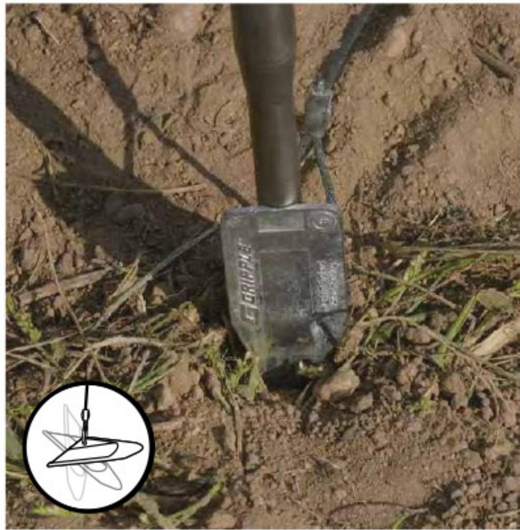
Anchor 3 - Being driven into the ground.
